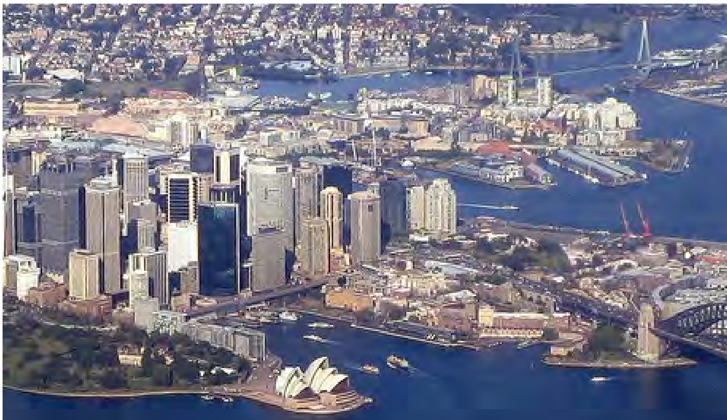
Central Sydney / The Rocks Conservation Area
