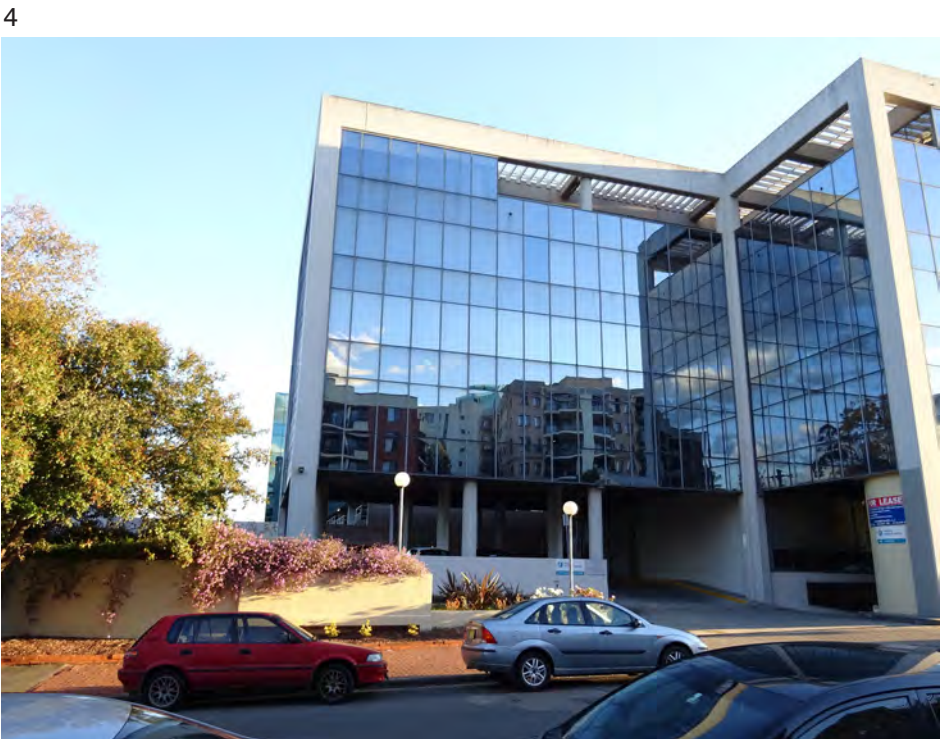
4 storey commercial building located immediately to west of Site.
