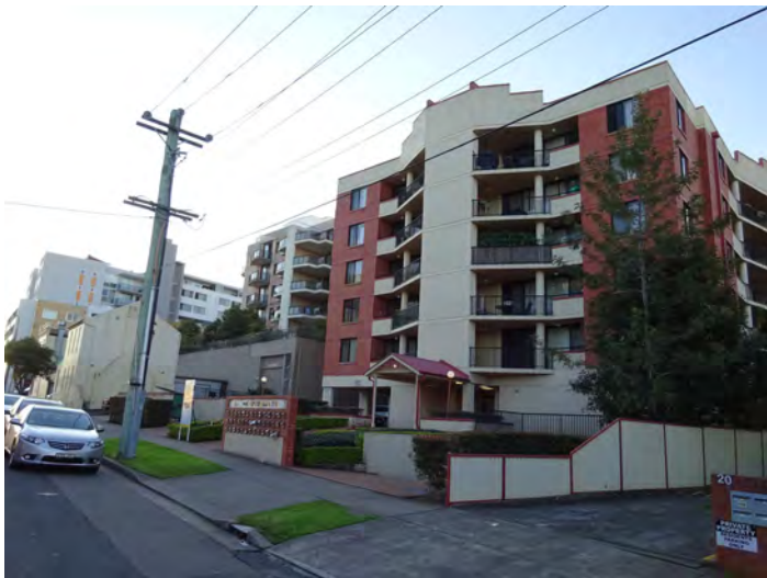
6 storey residential flat building located on Harold Street.
